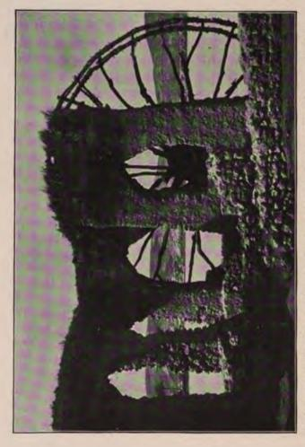
Modern water wheel or na'ura in Babylonia. The river is dammed up and the water made to pass the wheel to which, when in use, paddles were attached and bottles to lift the water to the aqueduct.
